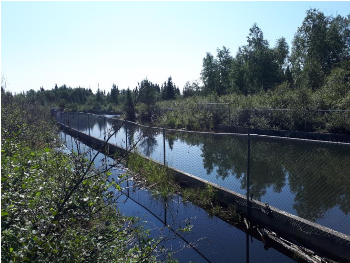
Figure 12-1: Flooded glory hole on Robitaille mine, Chapais, Quebec
